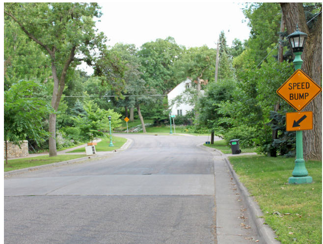
Speed hump locations are often indicated with signage to further alert drivers to slow speeds.
