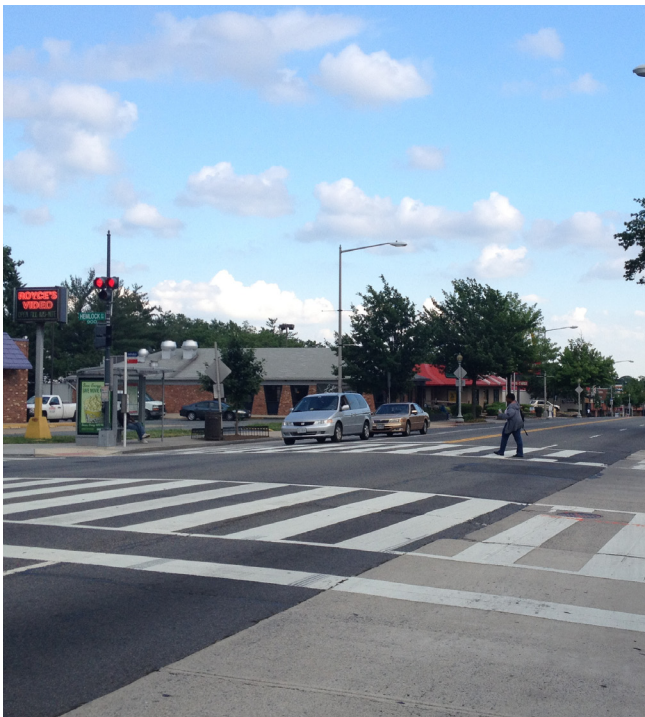
Ladder style crosswalks provide greater visibility for approaching drivers.
