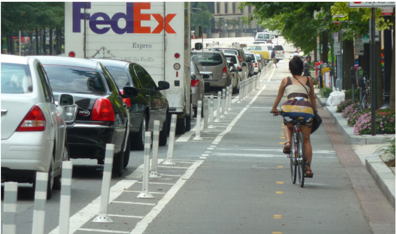
Cycle tracks can be designed to be two-way facilities on a one-way street. Signage and pavement markings are provided at driveway crossings to alert drivers to the presence of two-way bicycle cross traffic.
