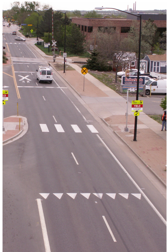
Advance yield markings on this multi-lane street alert drivers to expect pedestrian crossings ahead.
