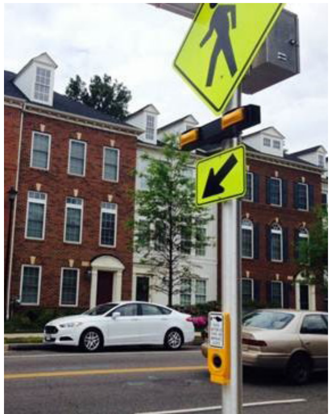
Push buttons are located on the sign post of the RRFB which must be supplied with an electrical connection.
