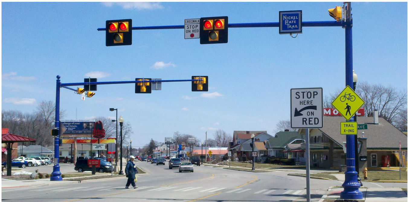
HAWKs are particularly useful in multi-lane contexts like the one pictured here where a multiple threat crash risk exists.
